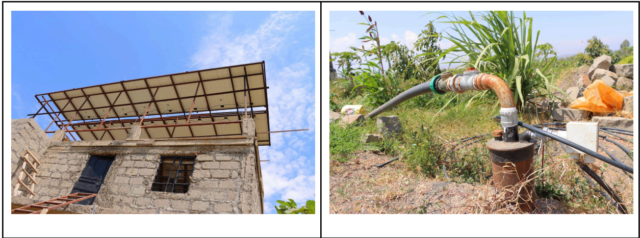
Figure 4: Installed solar-powered irrigation system at George's farm
