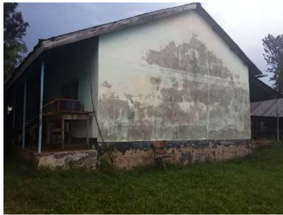
Proposed facility for BIH Occupation at Mabanga ATC. Rehabilitation required
