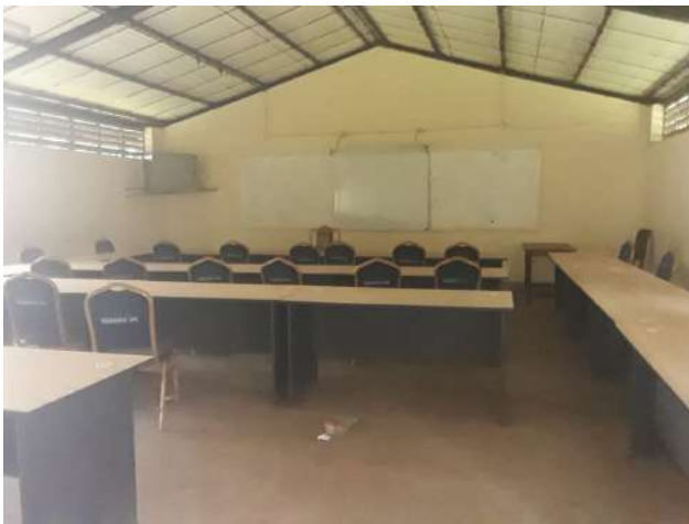
Mabanga ATC Classrooms
